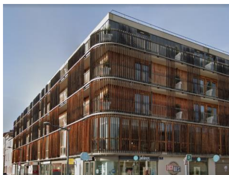
Photo 1: Dock Ouest ©Keys REIM
