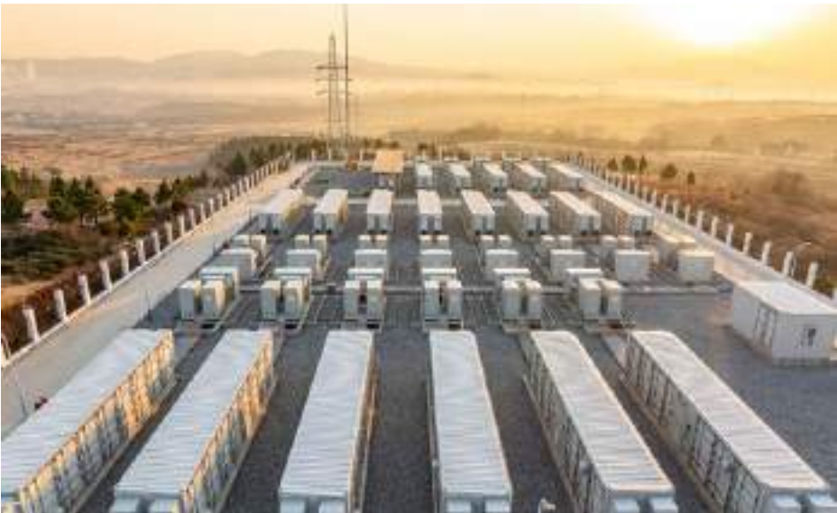
Power play Battery storage is in demand
